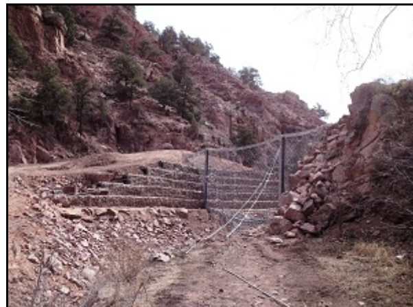
Fig 6. VX net (below) and UX net (above) with armored access abutment, Glen Eyrie Conference Center, Colorado Springs, Colorado.
