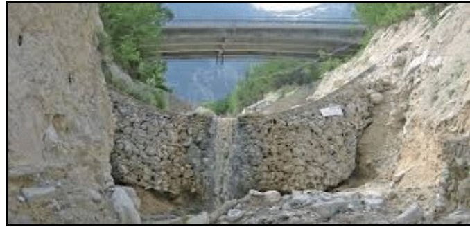
Fig 1. Instrumented test net in the Illbraben, Leuk, Switzerland.
