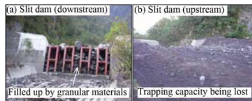
Fig. 1 Slit dam filled up by granular materials (the pictures from Shima et al., taken in Rishiri island, Japan, 2016)
