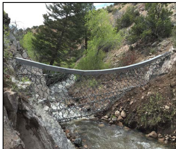
Fig 3. Post-fire VX net installed above running stream in Nambé, New Mexico. Note basal opening allowing water and fish passage beneath. Animals can pass either underneath or through rings.
