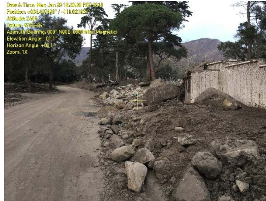
Fig. 5. View north of E. Valley Lane, approximately 150 meters south of State Route 192, showing the condition of cleared secondary roads at the time of the GEER reconnaissance.
