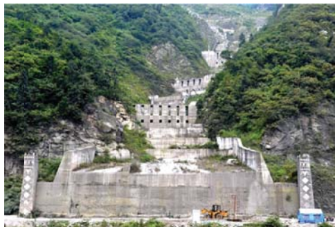
Fig. 3 Cascade check dams with orifices of various sizes in Shaofang gully, China
