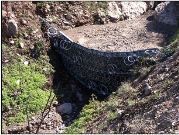
Fig 9. Filled VX debris net in Camarillo, California.
