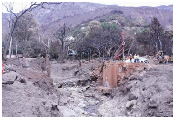
Fig. 9. Abutments of former East Mountain Road bridge at San Ysidro Creek, January 30, 2018. Burned vegetation due to fire associated with gas line explosion.
