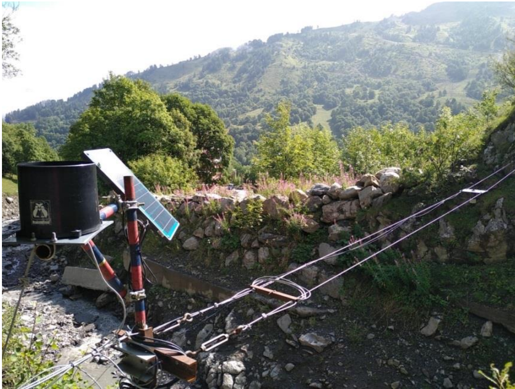
Fig. 6. Flow monitoring station located at the fan apex (pink dot in Fig 1.b) with: rain gauge, solar panel and flow stage sensor on cables; all devices are connected to a datalogger.
