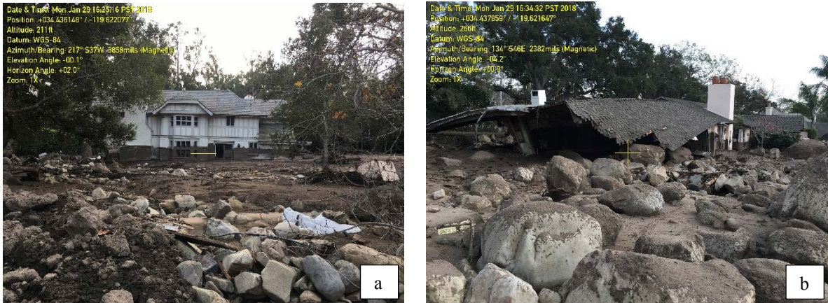
Fig. 11. (a) accumulated debris flow deposit and intact structure on East Valley Lane approximately 360 meters downstream of the point of debris flow avulsion from San Ysidro Creek channel at SR 192 bridge and 277 meters due west of the San Ysidro Creek channel. Note prominent mudline, this home was located along the western margin of the debris flow deposit. (b) accumulated debris flow deposit and partially destroyed structure on East Valley Lane approximately 165 meters downstream of the point of debris flow avulsion from San Ysidro Creek channel at SR 192 bridge and 135 meters due west of San Ysidro Creek channel. This home was located within the direct flow path of the debris flow after the flow overtopped the San Ysidro Creek channel.
