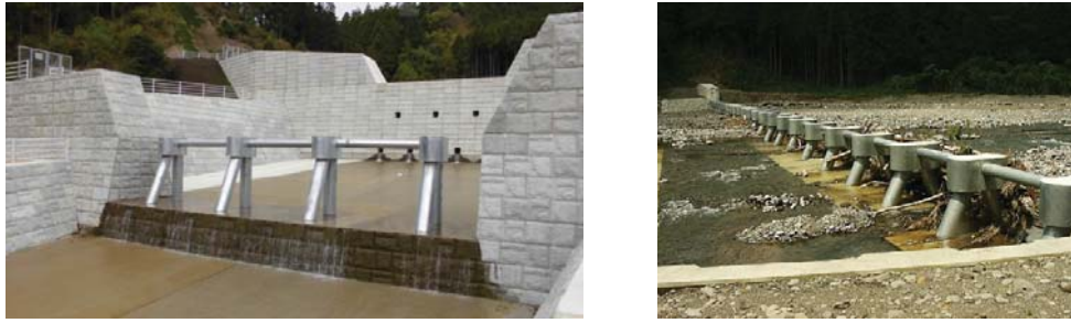
Fig. 2. Sub-dam with stakes installed near the foot of the Sabo dam
